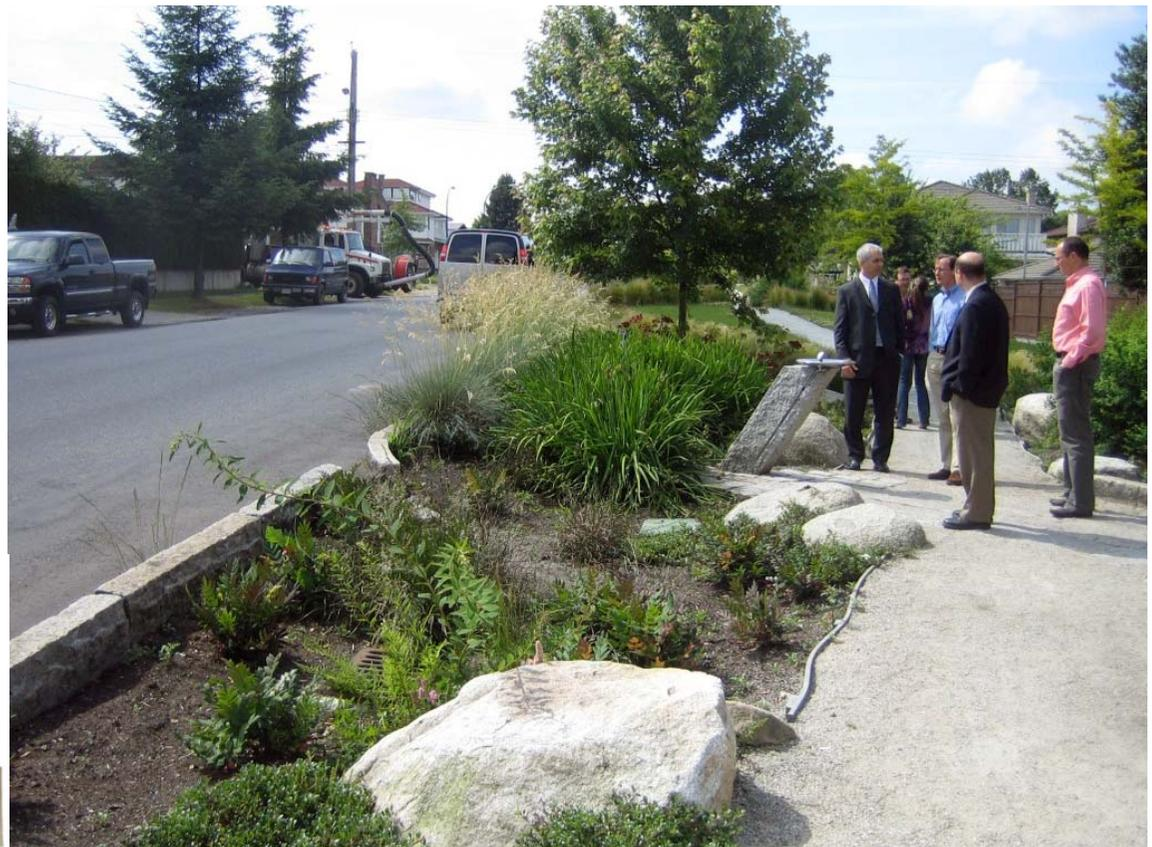
Water flowing off impervious surfaces (for example a roof or driveway) can be delivered to the rain garden through a swale lined with decorative rock or plants, through a pipe, or across a landscape area.
